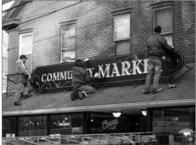
Sign installation at the D&D Community Market. Photo by Phyllis Segura
