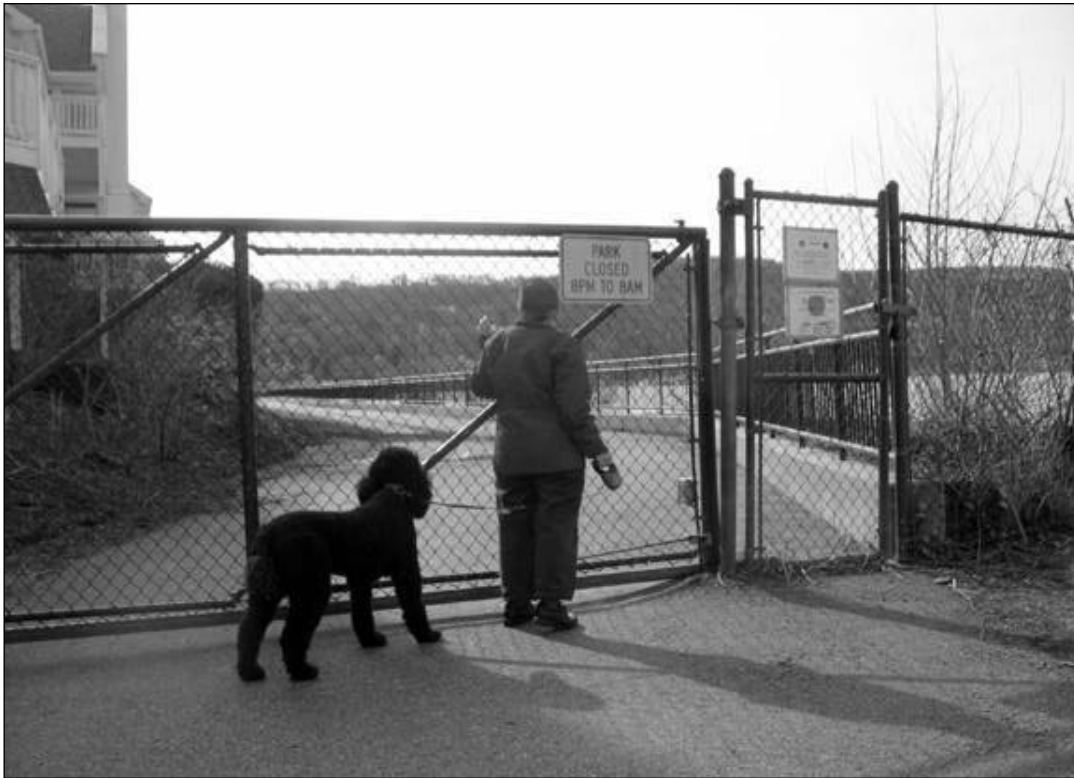
A dog walker was surprised to find the pier's North Shore Walkway closed for repairs. It has since been reopened. Bob Samuels photo
