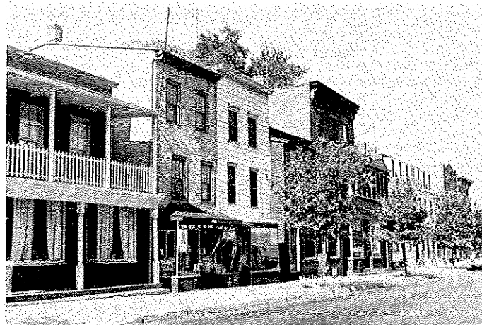
West Side of Main Street Looking North
