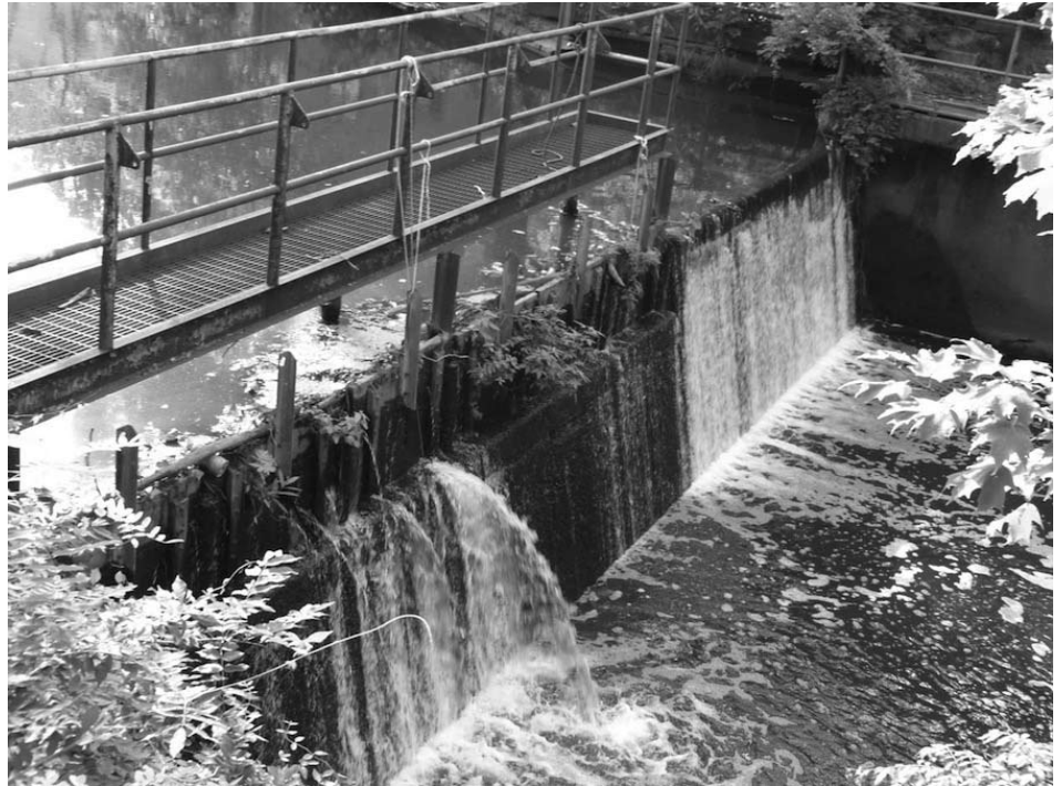
Dam on Sparkill Creek at Rockland Road Bridge. Ron Derven photo
