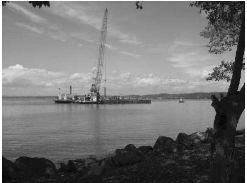
Channel markers being set into place Photo by Bob Samuels
