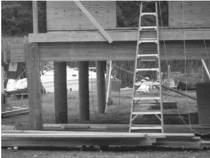
Home construction on Paradise Avenue. Fred Burrell photo
