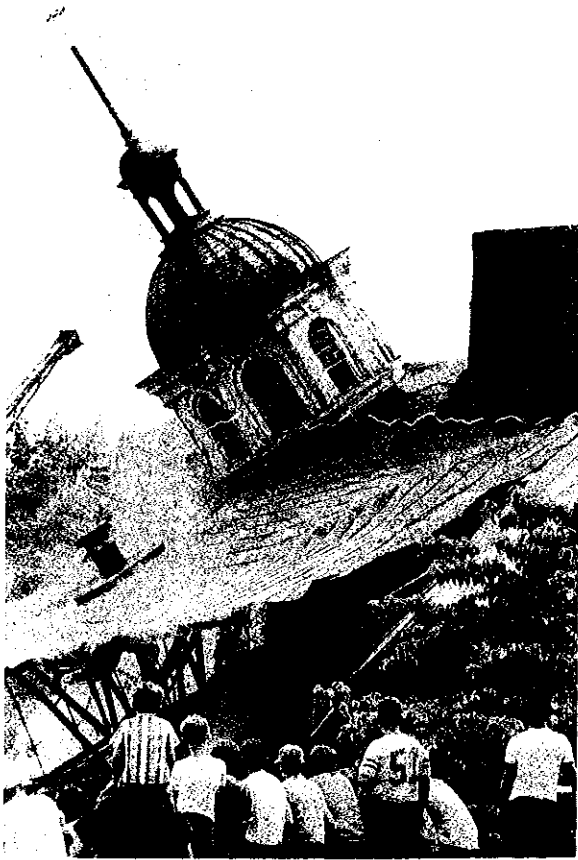
July 29th -- Demolition Day
